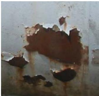
Preparation is a very important step in the painting process. The length of time paint adheres to a surface is often in direct proportion to the extent of preparation.
