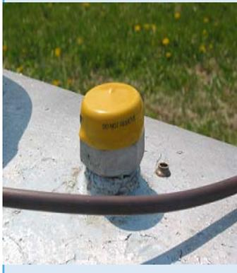
bris can clog the weep hole. If the weep hole cannot be unclogged, the valve should be replaced.
